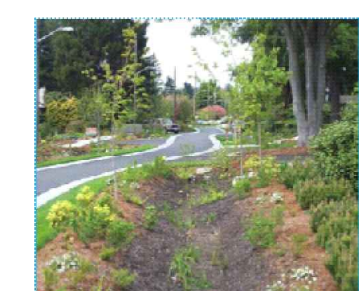
LID SWALE ALONG PEDESTRIAN PATH
